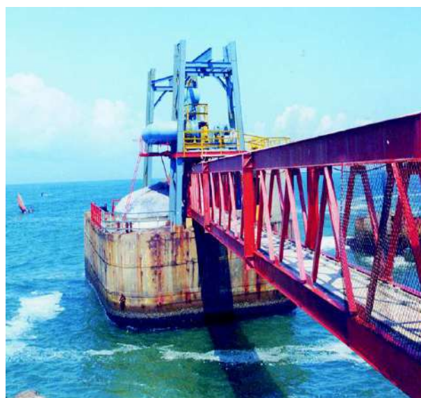
Fig. 6: Wave energy power plant at Vizhinjam. Source: Ravindran (1997)
