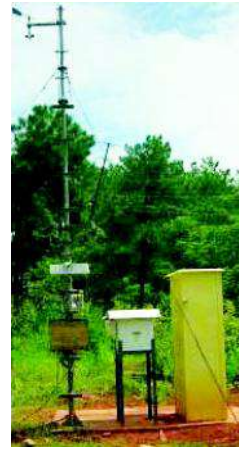
Fig. 10: Fuel cell power system installed by ISRO for powering automatic weather station at Shillong
